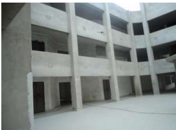
Plaster work almost completed of Main Building
