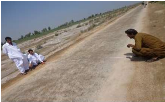
Width of carriage way is being checked in first mile
