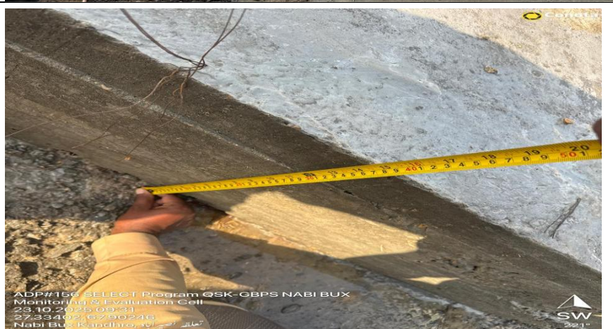
Measuring thickness of the RCC footing
