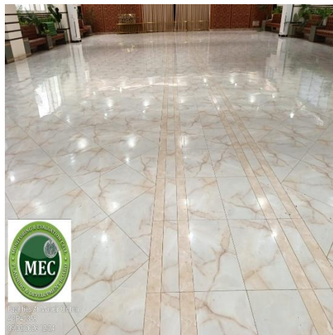
Glazed tile flooring and marble flooring.
